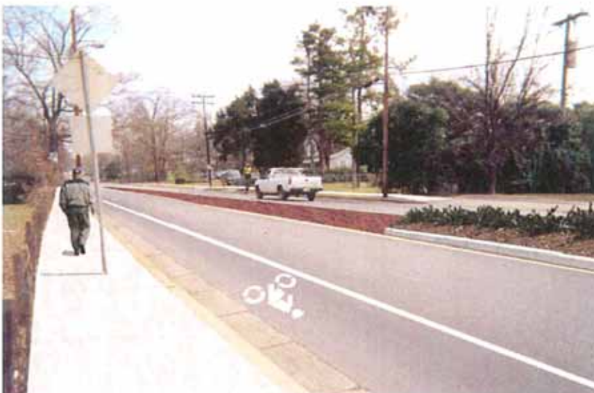
AFTER ROAD DIET: 2-Lane Road with Median, Bike Lanes, and Sidewalks
