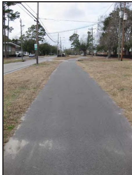
Colwell Avenue Greenway in front of Vesta Village
