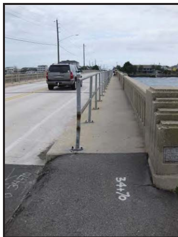
Existing sidewalk along Banks Channel Bridge
