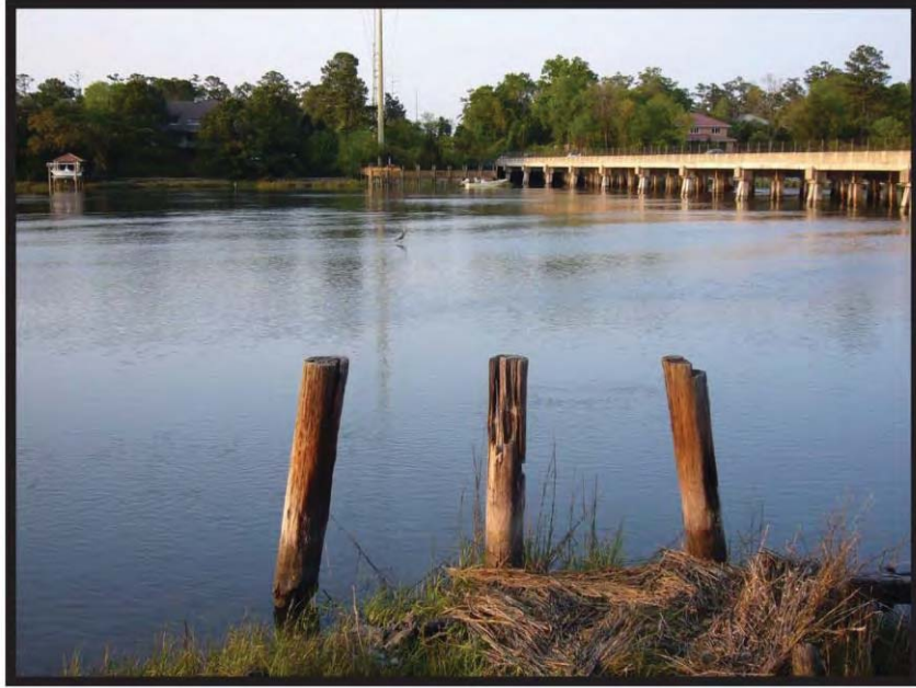
Terminus of Circular Drive at Bradley Creek
