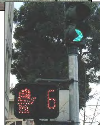
Figure 4-4. Example of a high-visibility crosswalk accompanied by a countdown pedestrian signal. A countdown pedestrian signal can be pedestrian-actuated if installed with the proper push button activation system.
