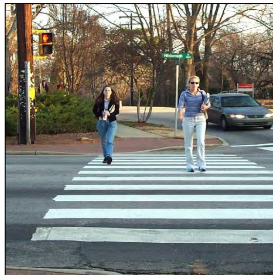
Figure 4-4. Example of a high-visibility crosswalk accompanied by a countdown pedestrian signal. A countdown pedestrian signal can be pedestrian-actuated if installed with the proper push button activation system.
