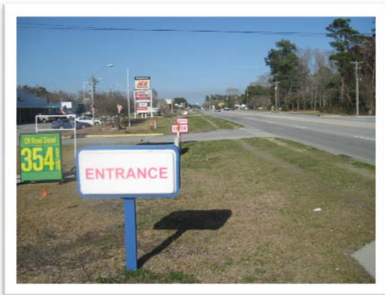
Multiple closely spaced one-way driveways may create driver confusion.
