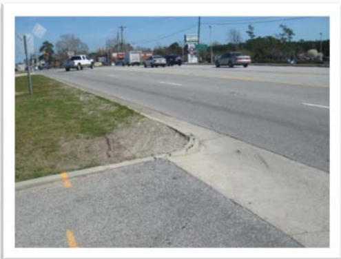
Small radius results in slower entering speeds and driving over the existing radius curbs.
