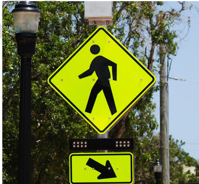
Figure 17: Rectangular Rapid Flashing Beacon
