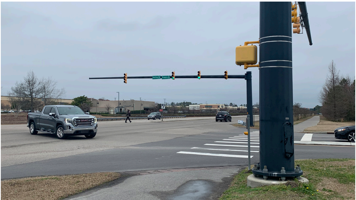
Sidewalk runs along Military Cutoff Road, but crossings of the major road are not provided at several intersections.
