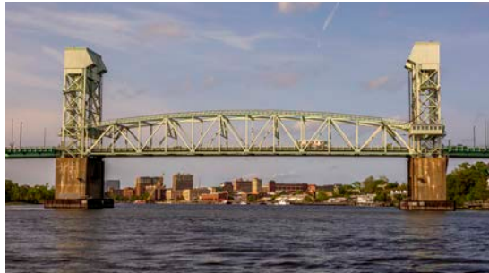
The Cape Fear Memorial Bridge.
