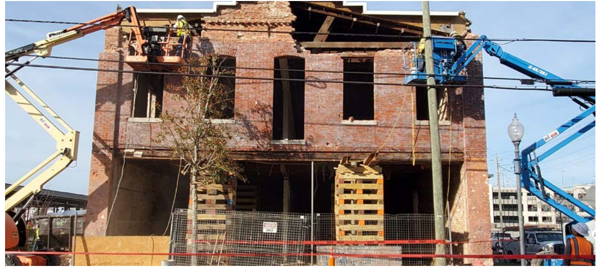
Building exterior work, February 2023.
