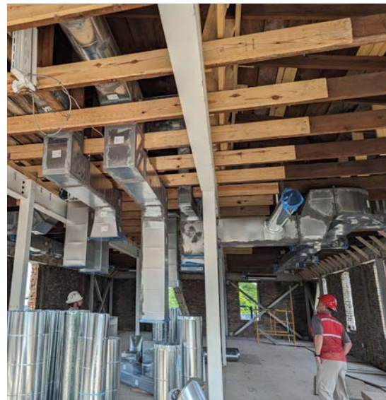
Building interior work, June 2023.
