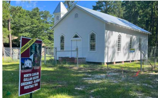
Reaves Chapel restoration site along the Gullah Geechee Heritage Corridor.
