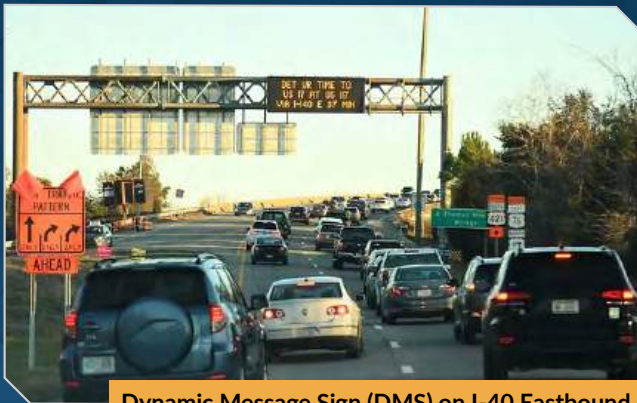
Dynamic Message Sign (DMS) on I-40 Eastbound
