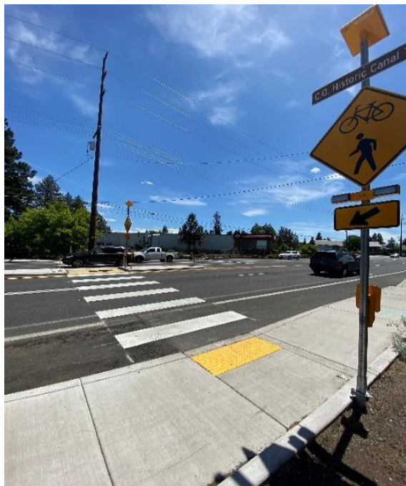
Figure 11: Crosswalk with RRFB (Above)
