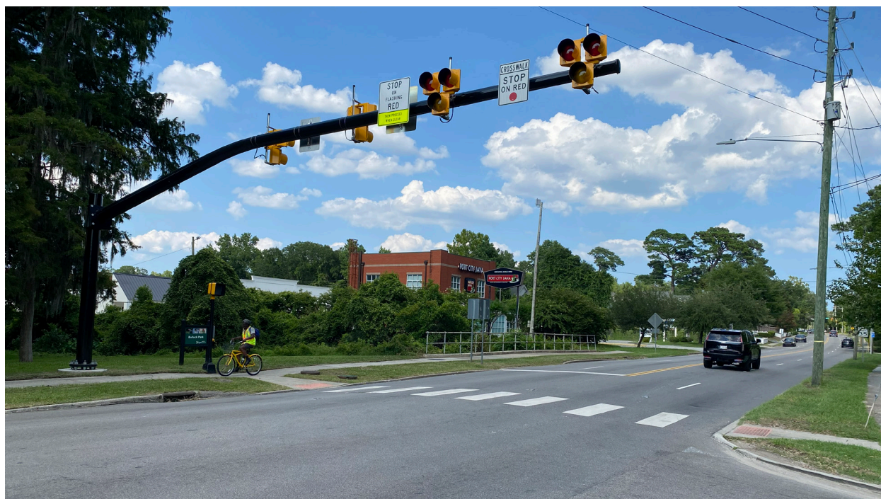
Photo credit: Kittelson. Pedestrian Hybrid Beacon on Market Street in Wilmington
