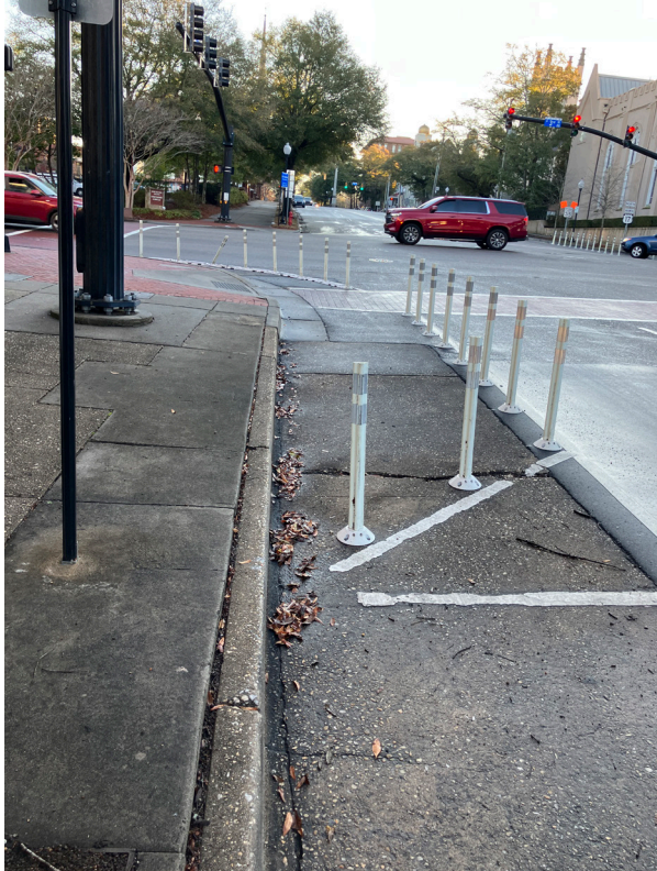
Photo credit: Kittelson. Quick-build curb extensions at Market Street and 3rd Street.
